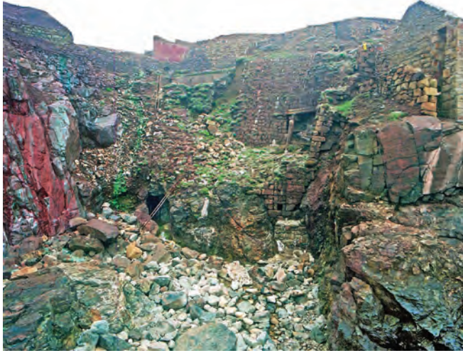
The drainage adit in the cliff face in 1991. The adit is at a slightly lower level 3 in Victory Shaft. The adit is now securely gated. Photo Nick Catford
